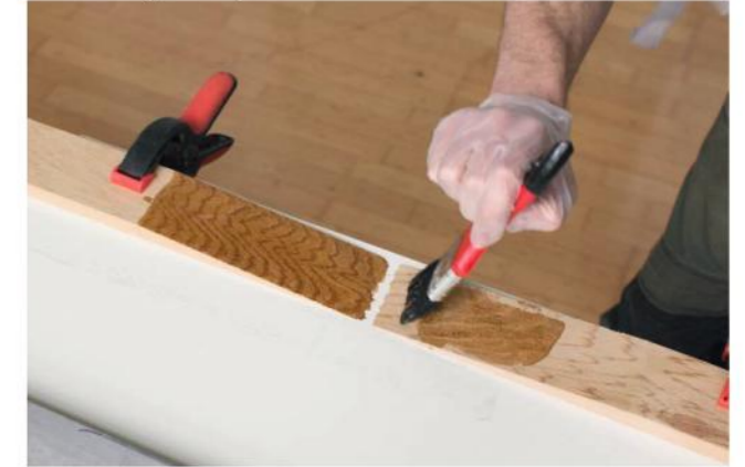
4 - Applying epoxy resin to the gluing surfaces
